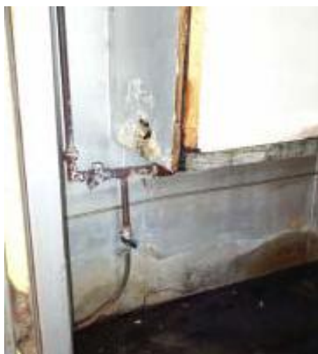
Figure 9.18 Leaking water lines
