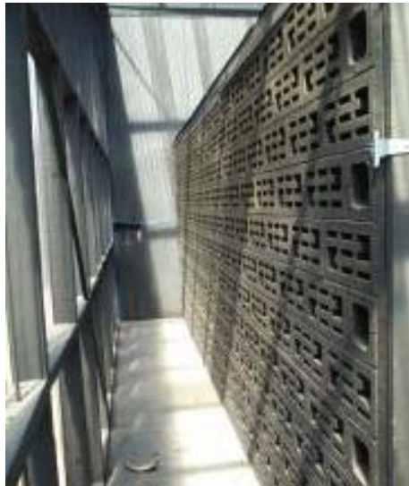
Figure 9.14. Breeze blocks provide thermal mass and an air diffuser in small greenhouse type unit
