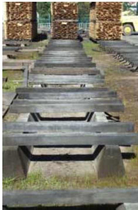
Figure 8.21. Fixed concrete kerb with bearers
