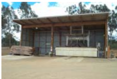
Figure 6.01. Fungicide treatment vessel and shed
