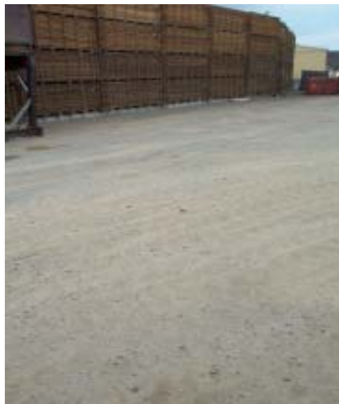
Figure 3.04. Firm and dry gravel hard standing
